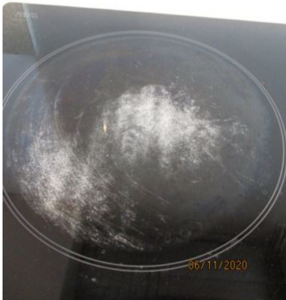
Image 39: LIVING ROOM AND KITCHEN hob ring badly marked
