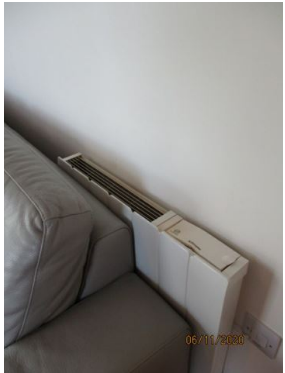
Image 30: LIVING ROOM AND KITCHEN
