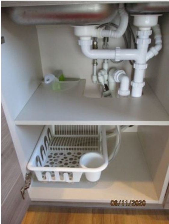
Image 37: LIVING ROOM AND KITCHEN
